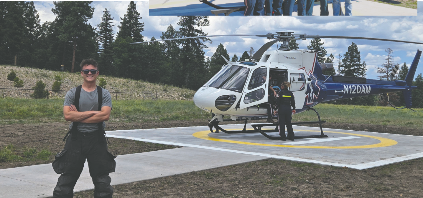
The new emergency medical helipad on Mescalero Avenue, dedicated in honor of Debbi McCurdy
