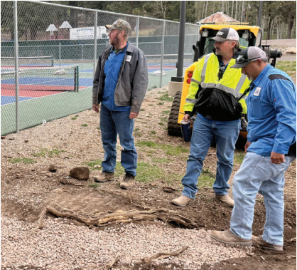
Public Works installs a French drain near the Zenith Park pickleball courts
